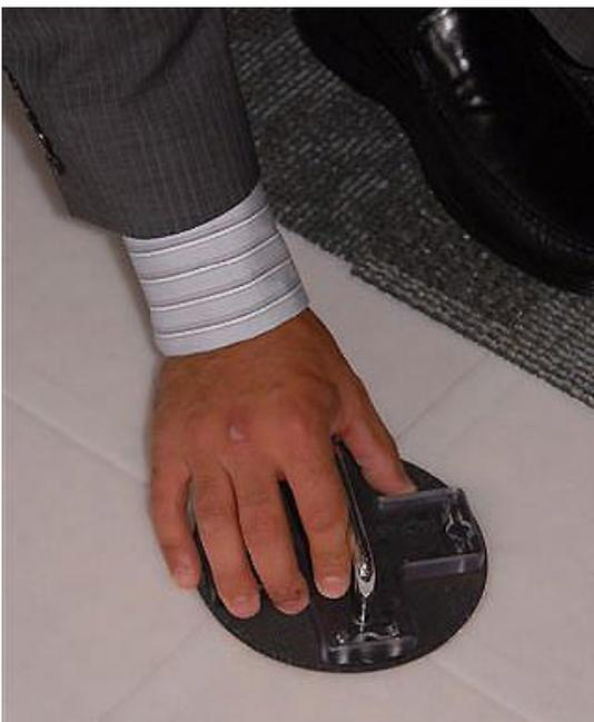
3. INSTALL AND LOCK OLACE CONNECTOR DISK
